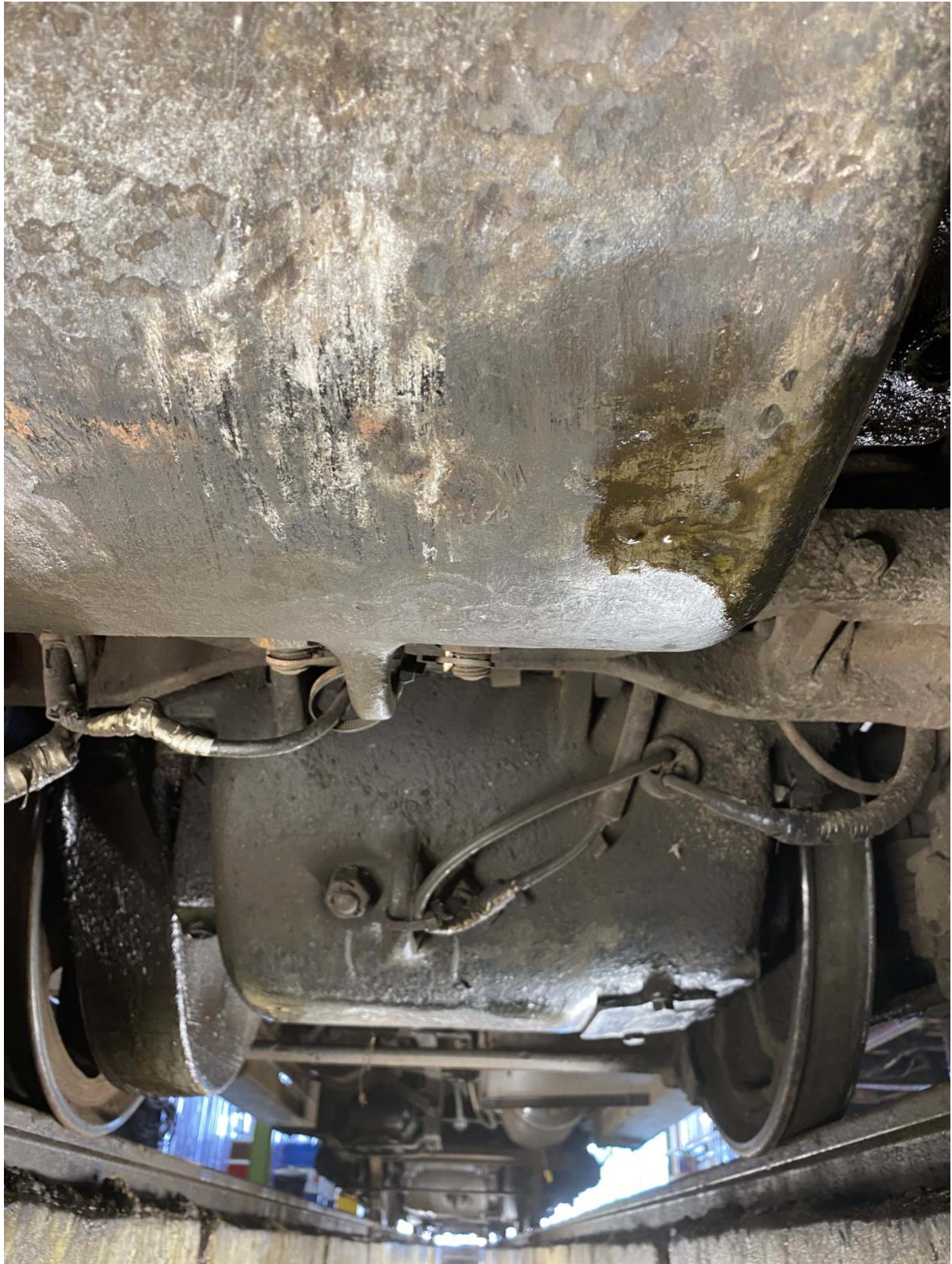
Marks on motor casing from contact with the rail head
