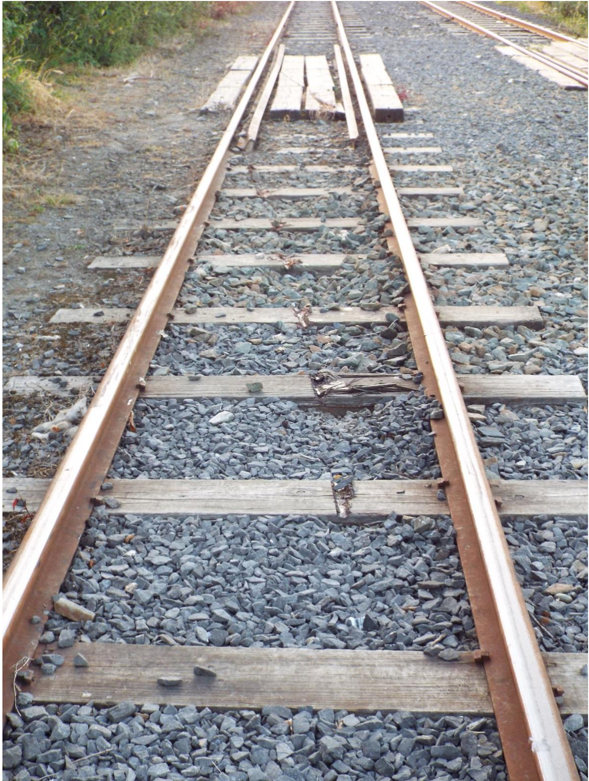
Right hand leading wheel contacted the check rails at the occupation crossing for Dreemskerry Farm. Second axle derails.
