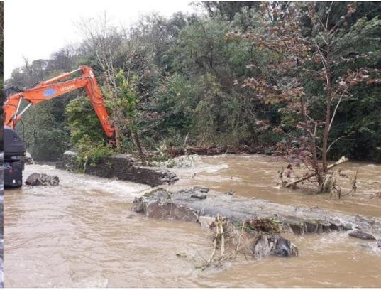
Photograph 6 - Collapsed wall during flood event (Gap B), nearside of wall is Glen Road.
