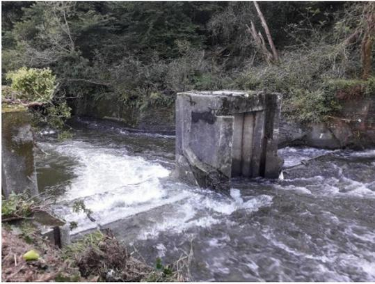
Photograph 7 - MER weir and sluice gate superstructure in the River Laxey, before removal.
