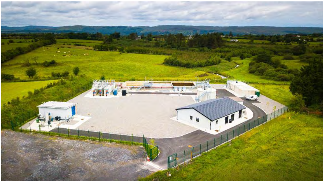
Figure 10: New treatment plant at Tubbercurry, County Sligo.
