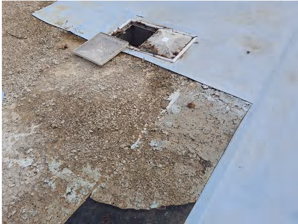
Issue 2: Spalled concrete top layer indicates freeze-thaw damage and moisture intrusion into basin structure.
