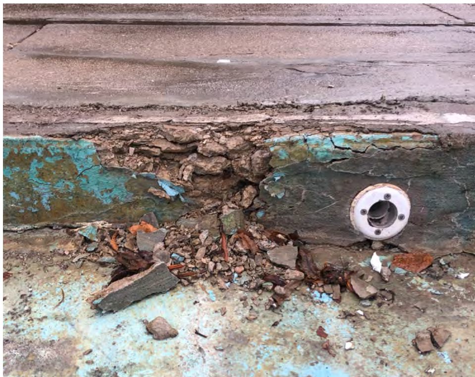
Issue 3: Damaged curb at curved zero-entry edge of pool
