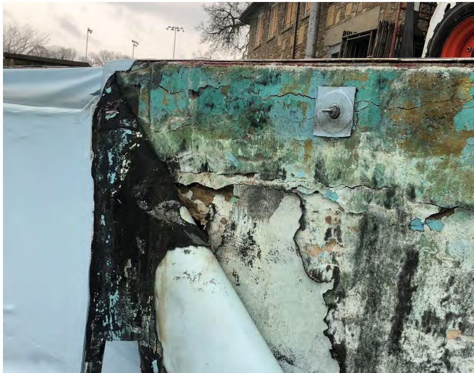
Issue 1: Cracks and spalling at North wall of pool indicate potential loss of integrity.
